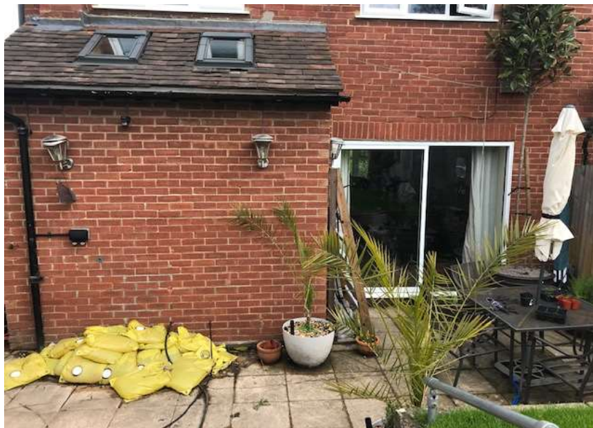
View of existing rear elevation and patio of application property
