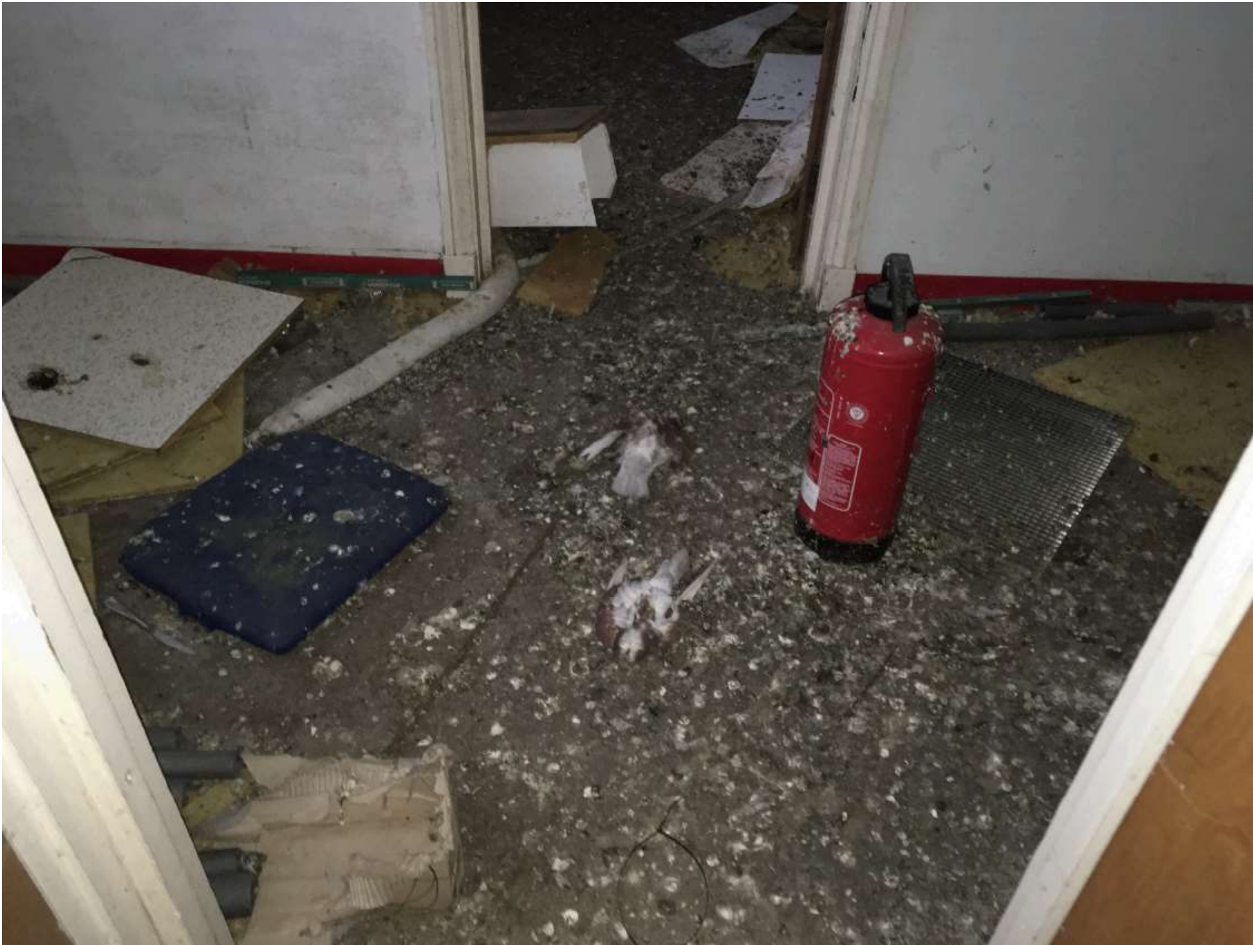
Image showing the internal condition of the building - image 3
