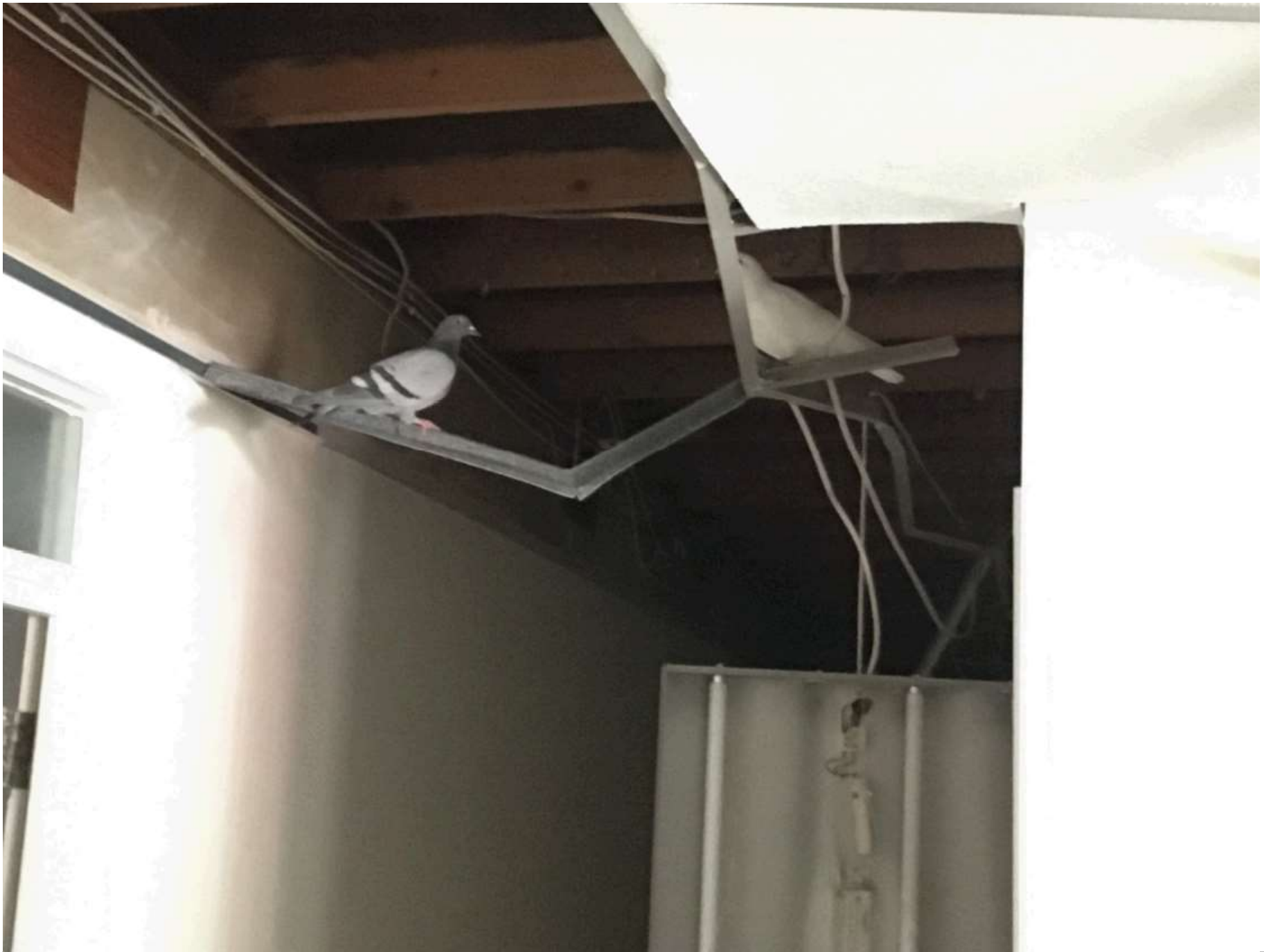
Image showing the internal condition of the building - image 5
