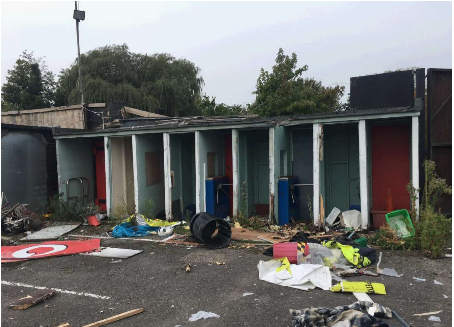
View of the turnstiles to be demolished
