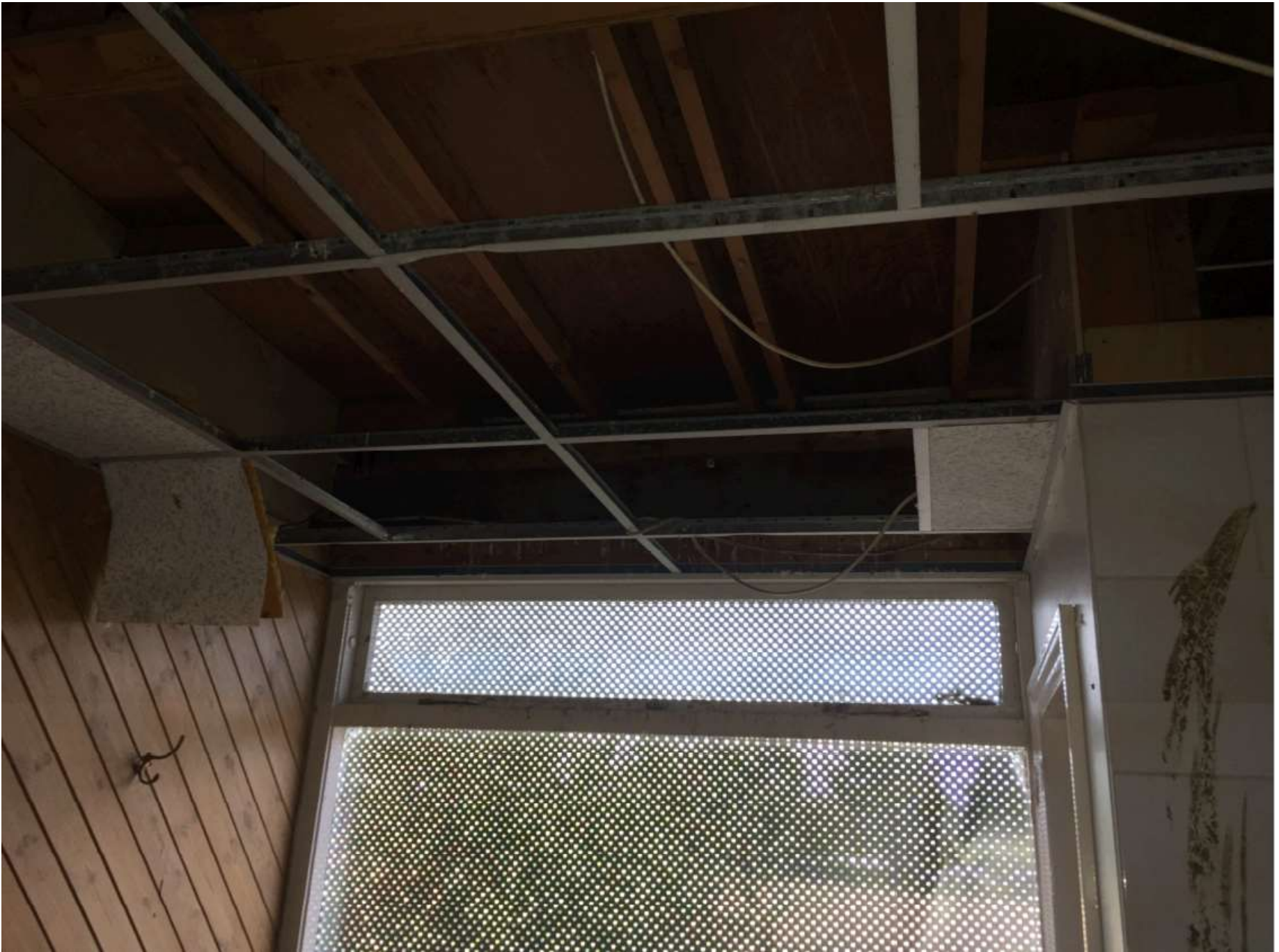
Image showing the internal condition of the building - image 4
