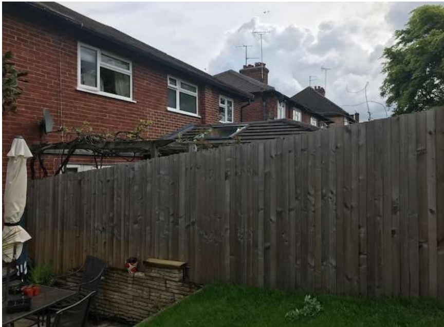
View of no. 3 Croft Road from rear garden of application site
