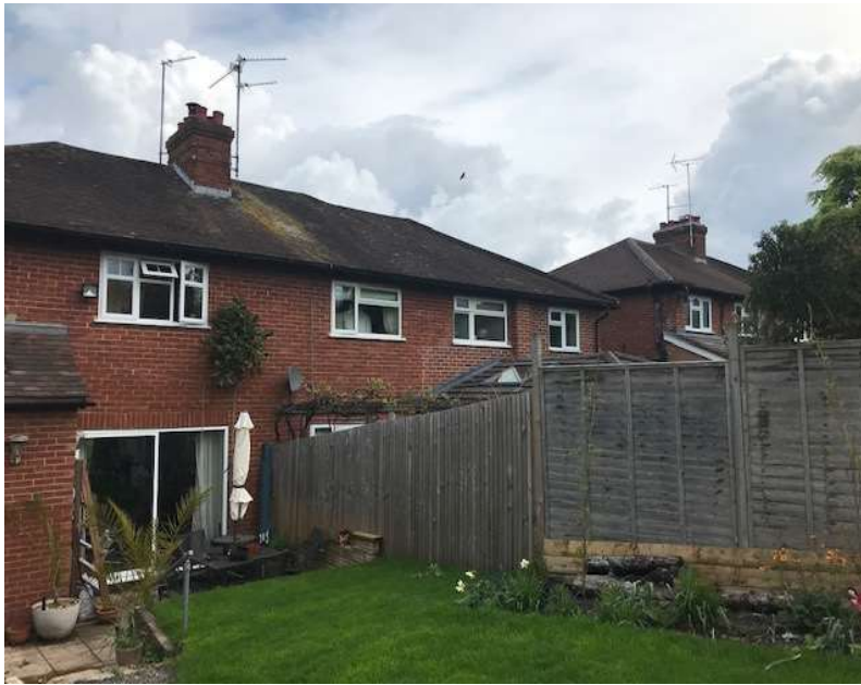
View towards no. 3 Croft Road from rear garden
