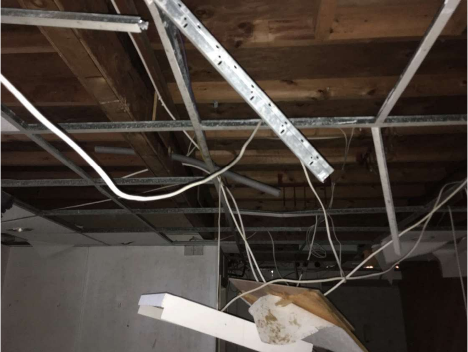
Image showing the internal condition of the building - image 2
