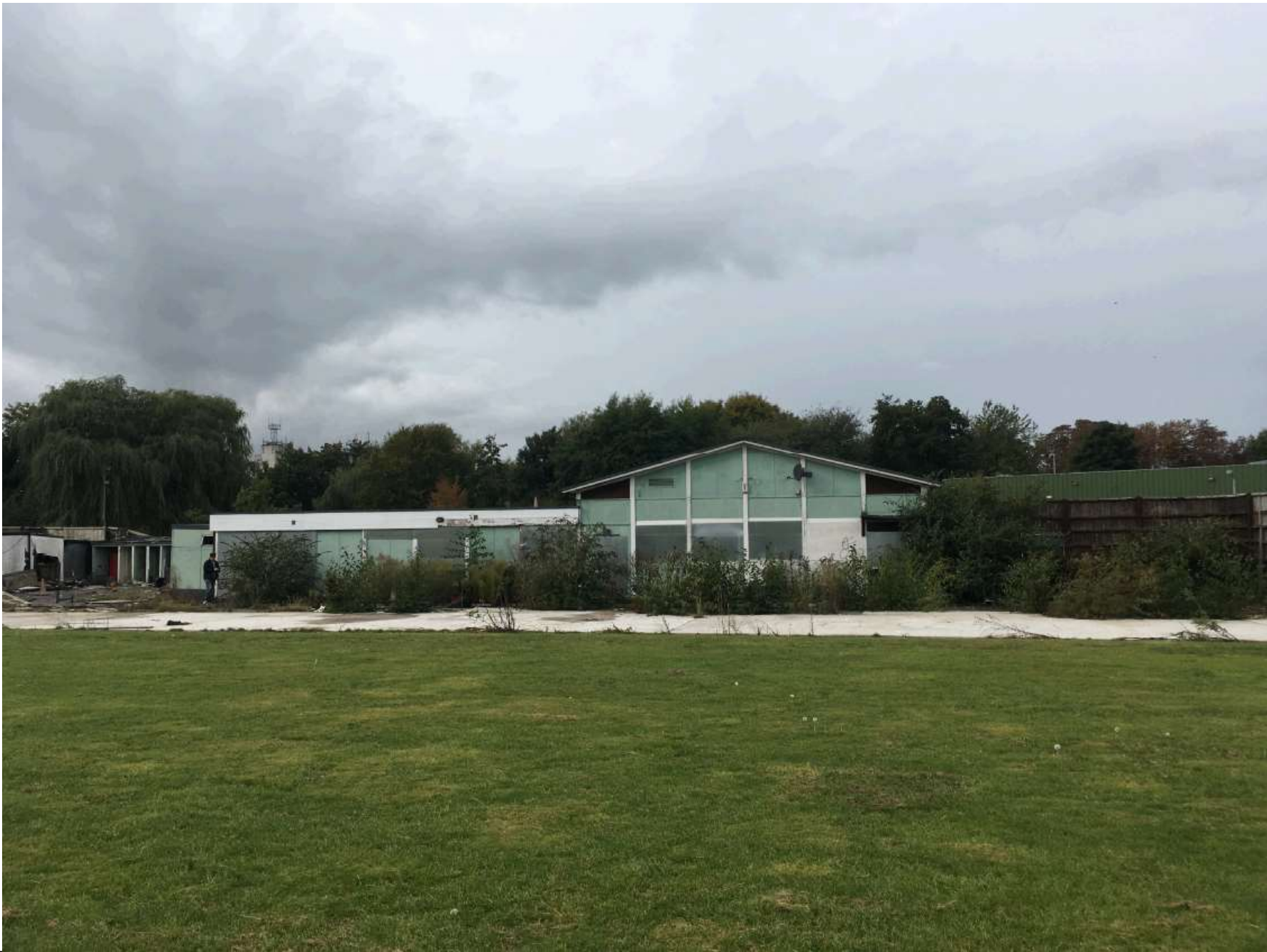
View of the clubhouse from the playing pitch looking towards the west. Also shows the hardstanding area left following the removal of the stands.
