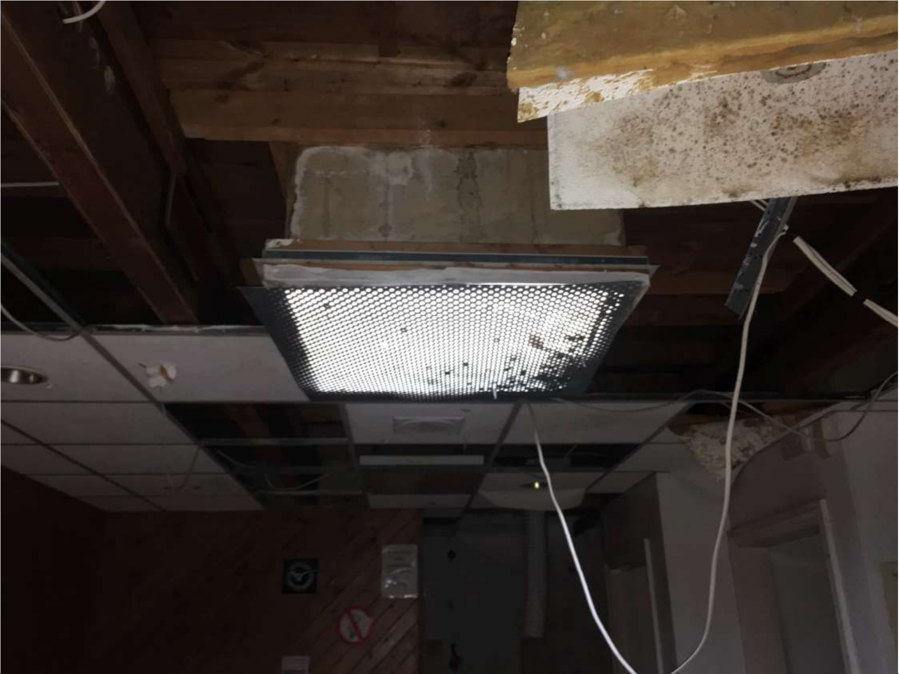
Image showing the internal condition of the building - image 6
