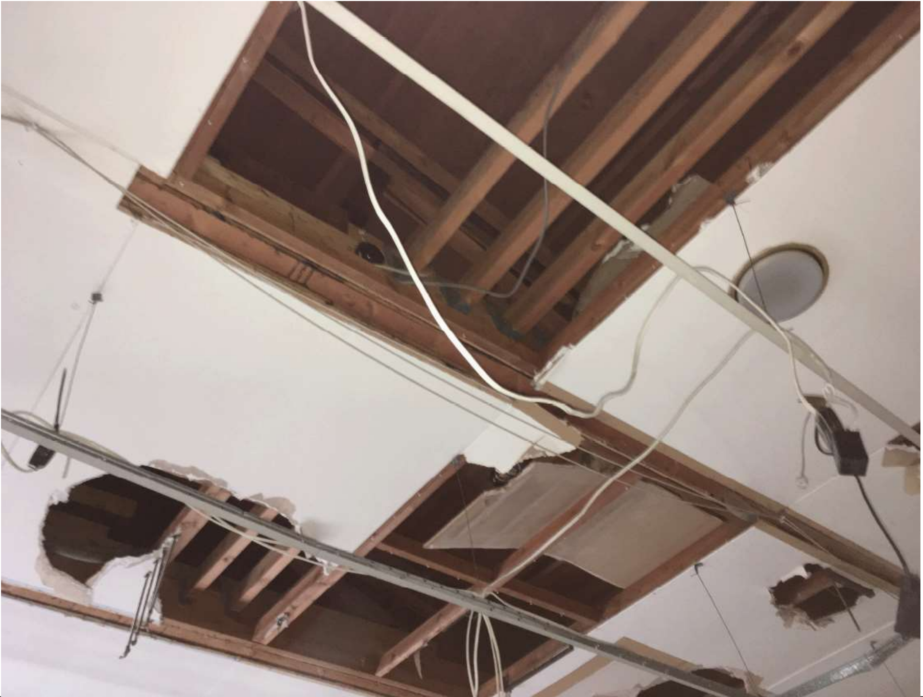
Image showing the internal condition of the building - image 7
