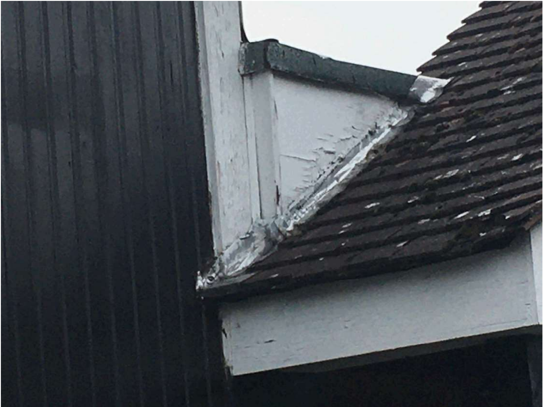
Image showing the condition of the building and its tiled roof
