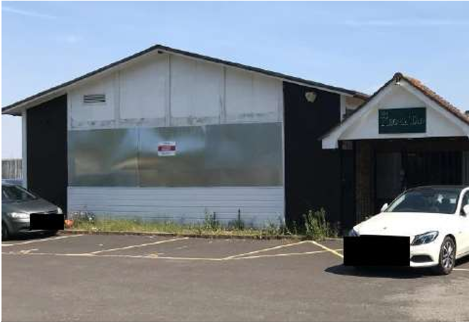
View of the clubhouse within the car park from the west looking east
